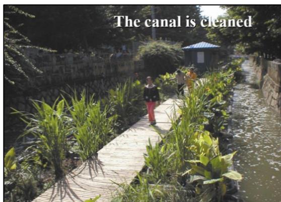
*Plate 8.5 Application of PhytoRid system to clean Nallah water*
