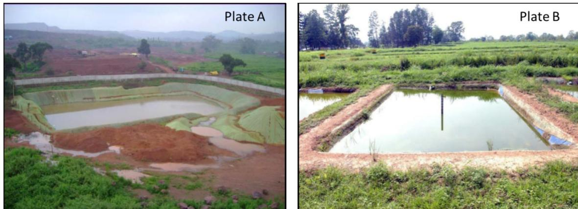
*Plate 8.10 (A and B): The Geogreen blanket used for protecting the slopes and base of the storage tanks dug on the ground to store rainwater (Courtesy: Sri Venkateshwara Fibre Udyog, Bangalore)*
