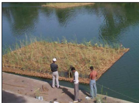
*Plate 8.6 Installation of Artificial Floating Island (AFI) in River Kshipra*
