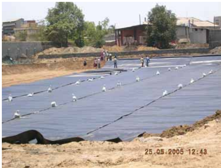
Secured Land-fill Work in Progress
