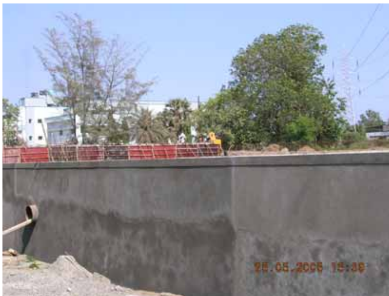
Construction of New 25 MLD CETP at Tarapur
